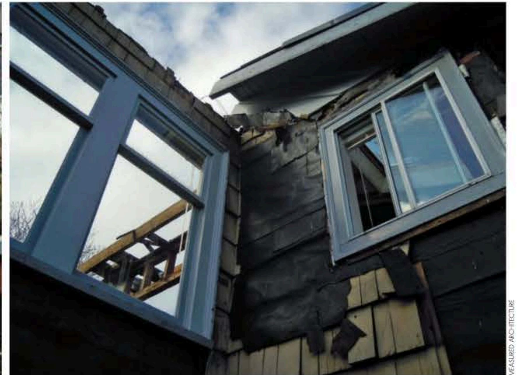
OPPOSITE TOP THE EXISTING DWELLING NECESSITATED DEMOLITION DUE TO ITS POOR CONDITION AND THE PRESENCE OF ASBESTOS. ABOVE, LEFT TO RIGHT SORTING THROUGH THE SALVAGEABLE MATERIAL; A VIEW OF THE PREVIOUS HOME AS IT WAS BEING DEMOLISHED.
